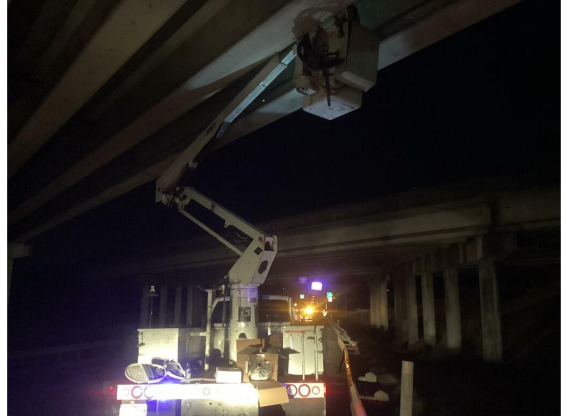
Loop 360 Underpass September 2023
